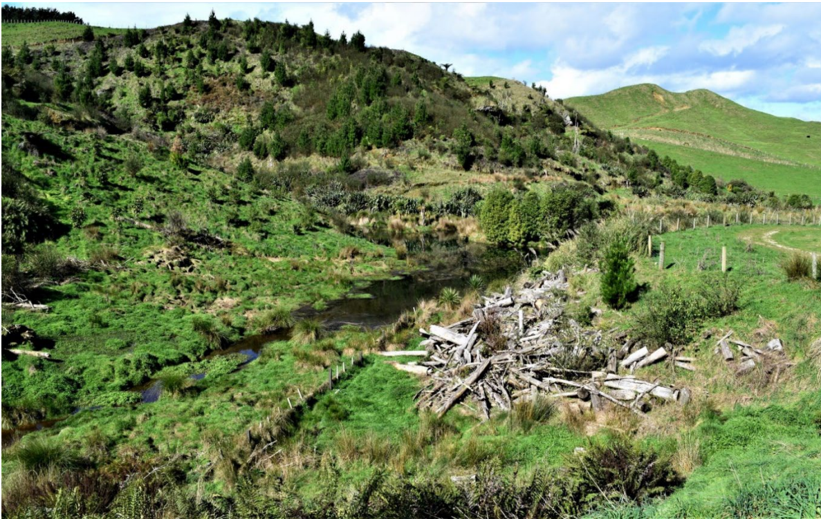
Main Dam gully August 2022
